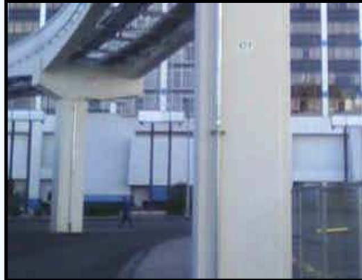
Massive support columns
