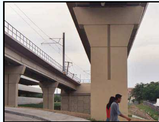
Massive support columns
