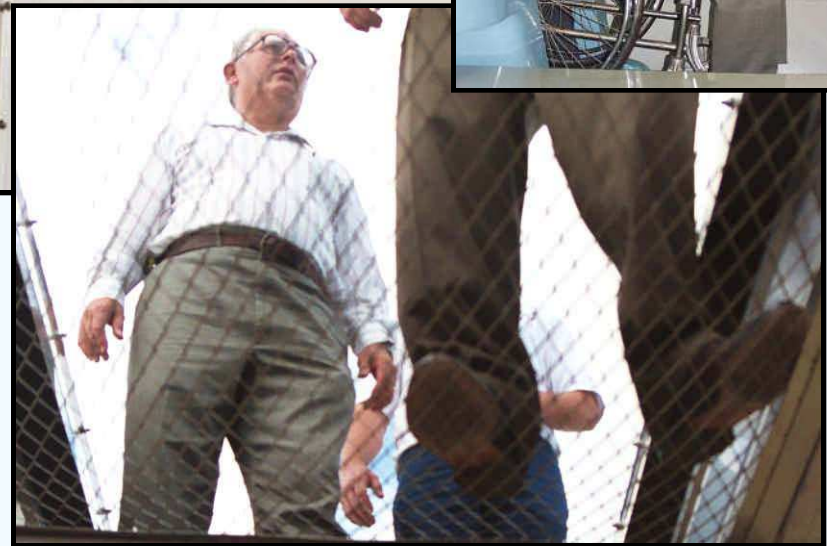
Upward view through walkway
