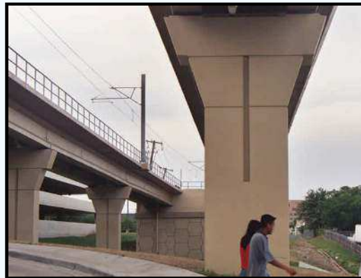
Massive support columns
