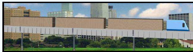
Elevated SuperWay electric operation
