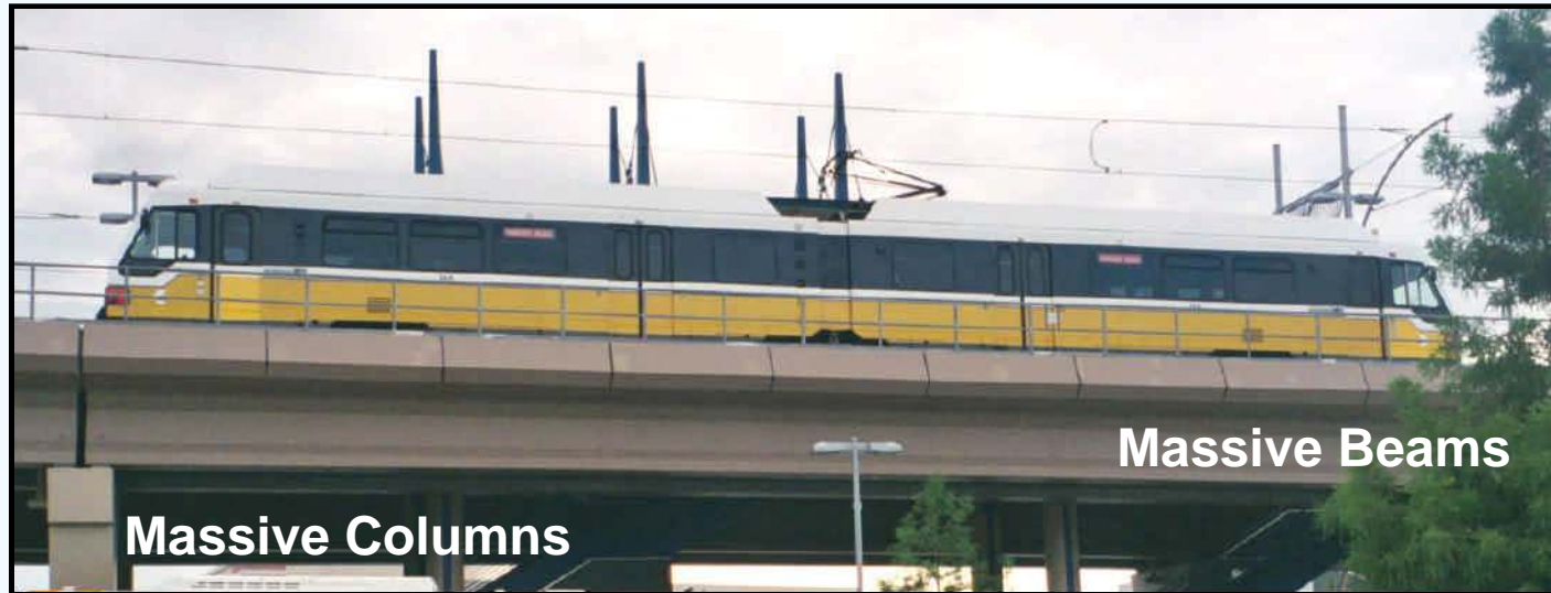
Elevated Dallas DART Light Rail Train
